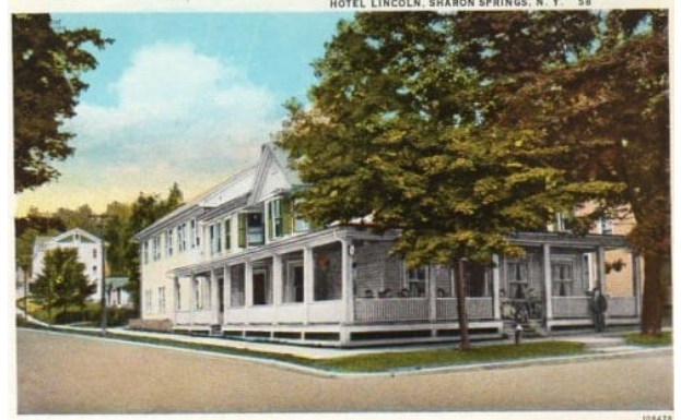
Lincoln Hotel at the corner of Main & South St. as it looked before it was damaged in the fire and then later remodeled.
