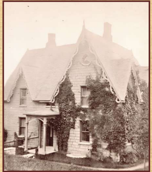
The same care and attention in construction and design was given to the Rectory as was given to the church.
